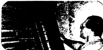
Drift eliminators can be removed for access to the prime surface coil
